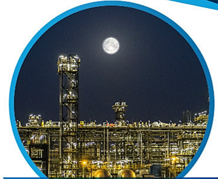
SHA GAS DEVELOPMENT (GASCO)
