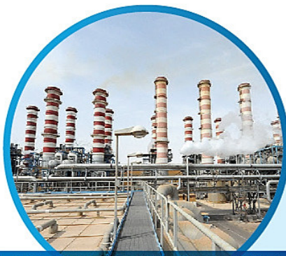
RAS ABU FONTAS DESALINATION PLANT (QATAR)
