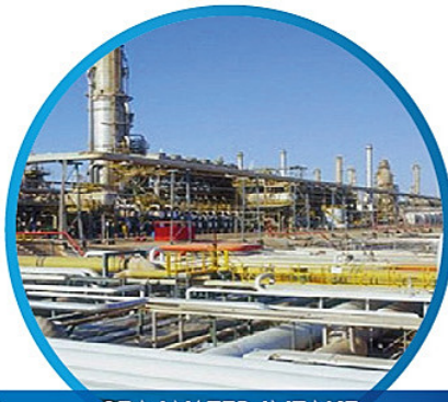
SEA WATER INTAKE PHASE III-RUWAIS (TAKREER)
